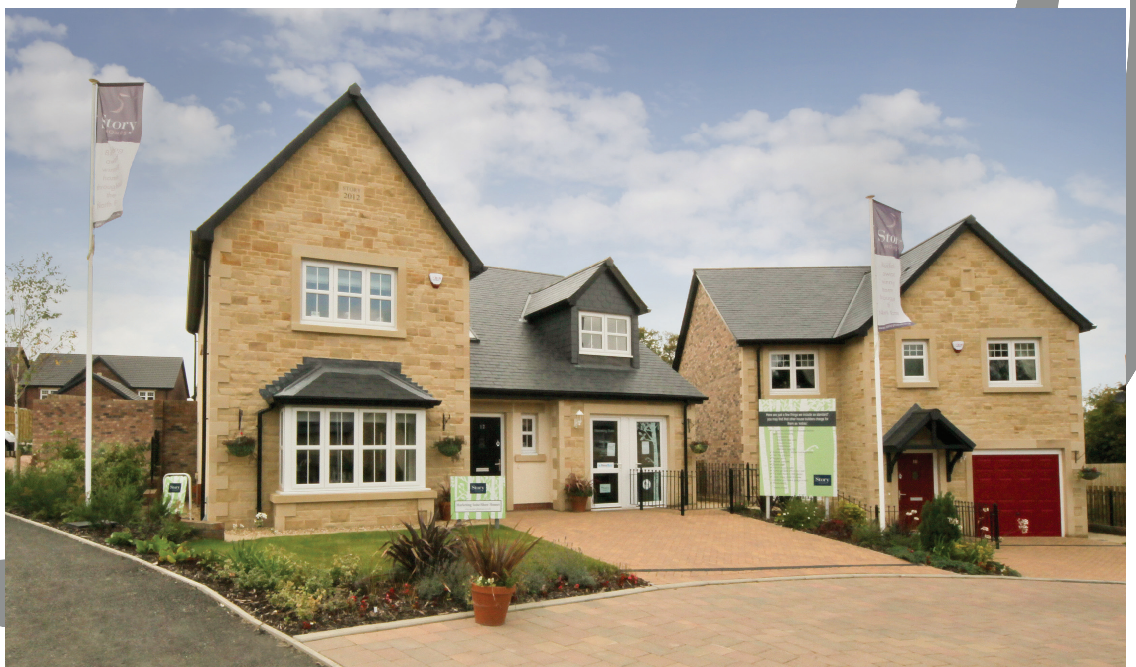
Award winning Story Homes development under construction at The Woodlands, Shotley Bridge
