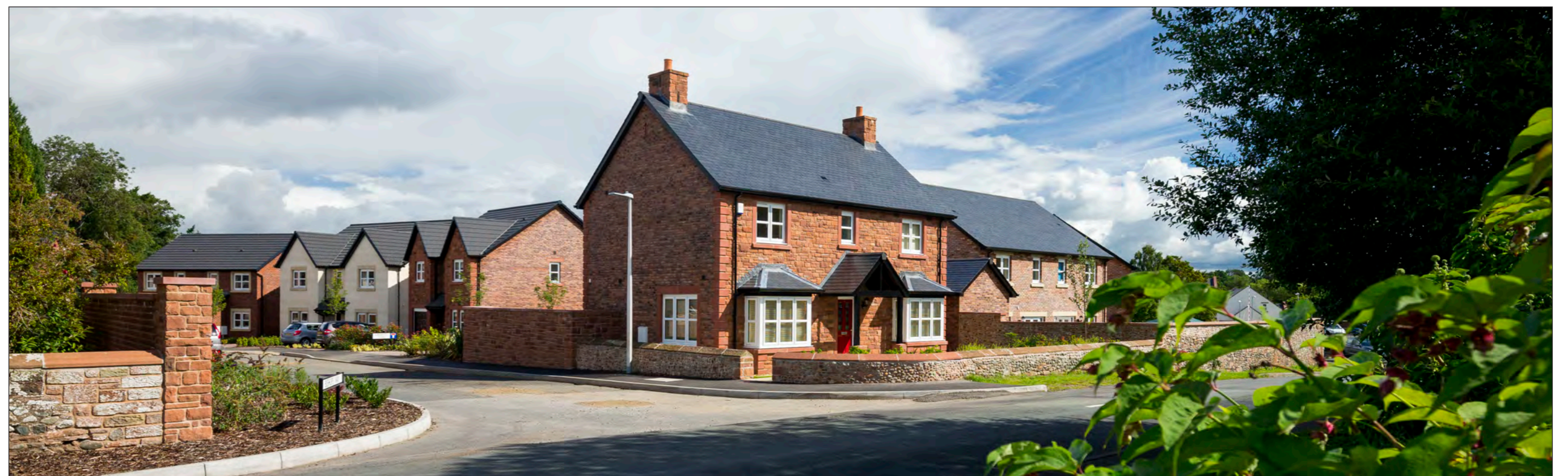
Story Homes development, Dalston, south of Carlisle
