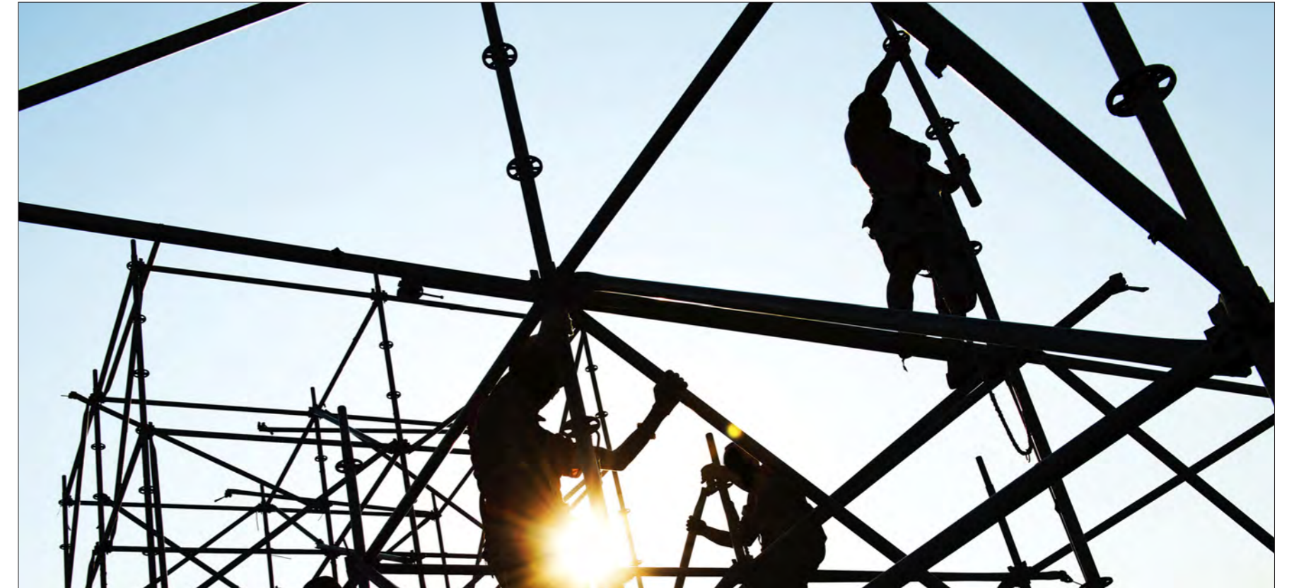
Story's construction team
