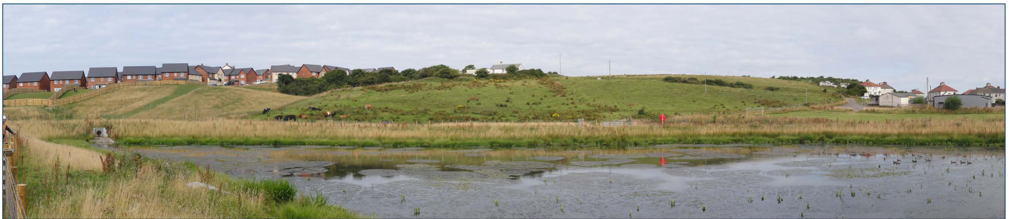
Extensive panoramic view looking west and north across the recently developed SUDS pond - introduced to deal with surface water drainage associated with Edgehill Park Phases II and III. Homes located towards eastern margins of Edgehill Park Phase II are visible to the left of this panoramic view. The proposed Phase IV site would be located between High House to the centre of the view and existing development at Valley View Road to the right. As part of wider proposals a new landscape buffer may be provided to the south of the proposed development which will help filter views through to any new homes alongside an extension to the existing pond and wetland area. This will be of benefit to local biodiversity
