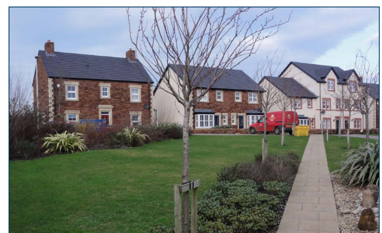
Initial Phases of Edgehill Park and wider development entrance off Wilson Pit Road
