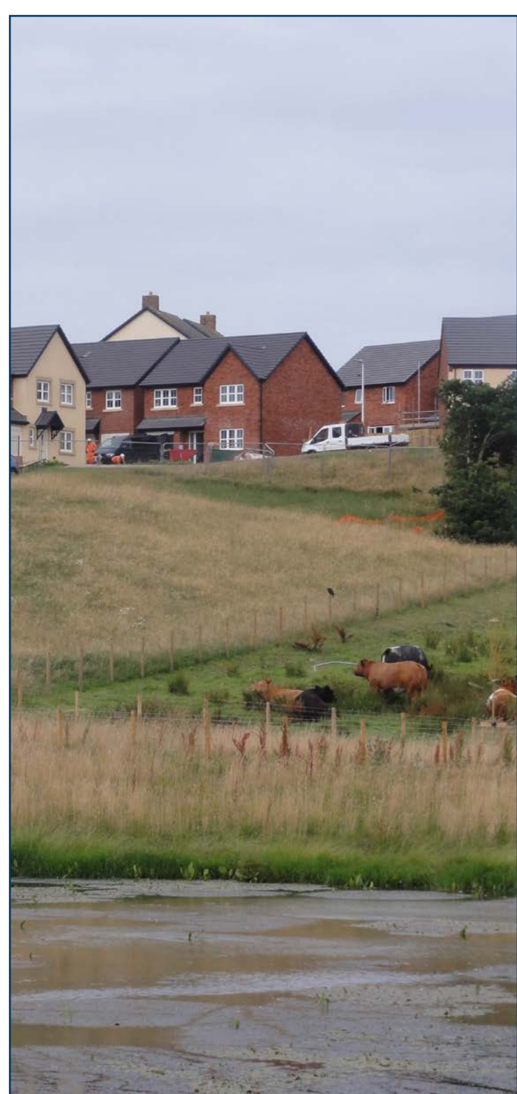
View looking across the recently developed SUDS pond - introduced to deal with surface water drainage associated with Edgell Park Phases II and III.
