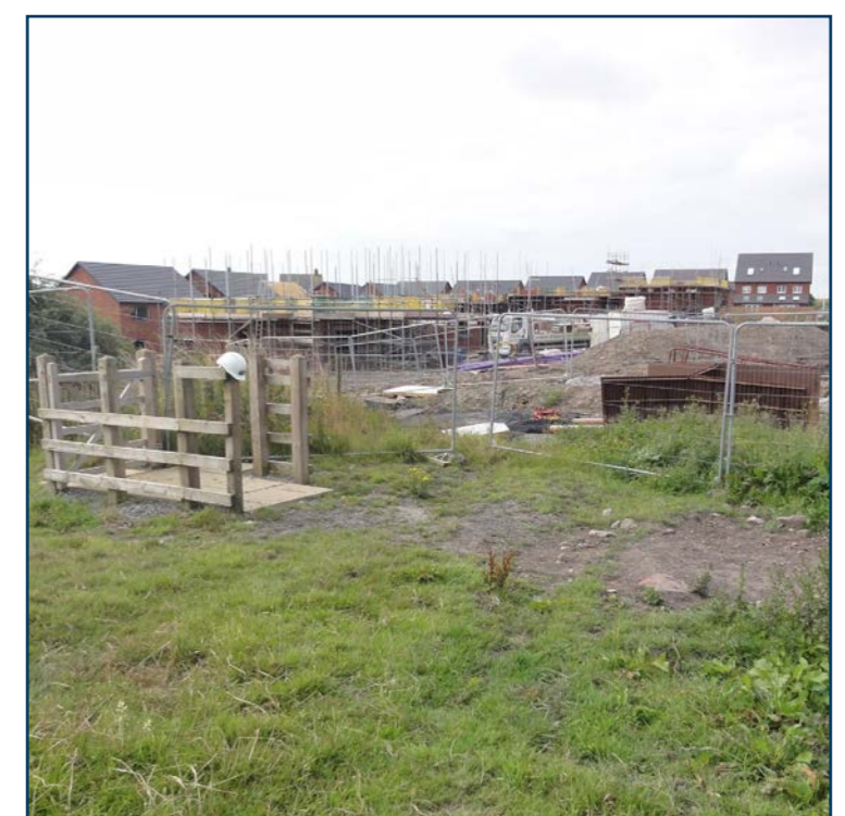
Edgehill Park Phase II under construction. The existing cross site PROW between Wilson Pit and Valley View Road will be slightly re-routed along attractive streets or through new open spaces
