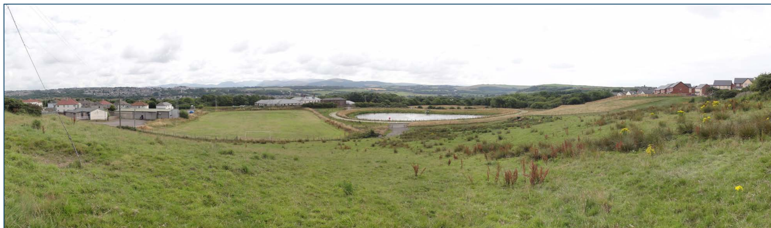
Panoramic view looking south from a point alongside the PROW / track to High House. Proposals may necessitate extension of the existing SUDS pond whilst there may also be opportunity to introduce new planting across existing slopes down to the feature
